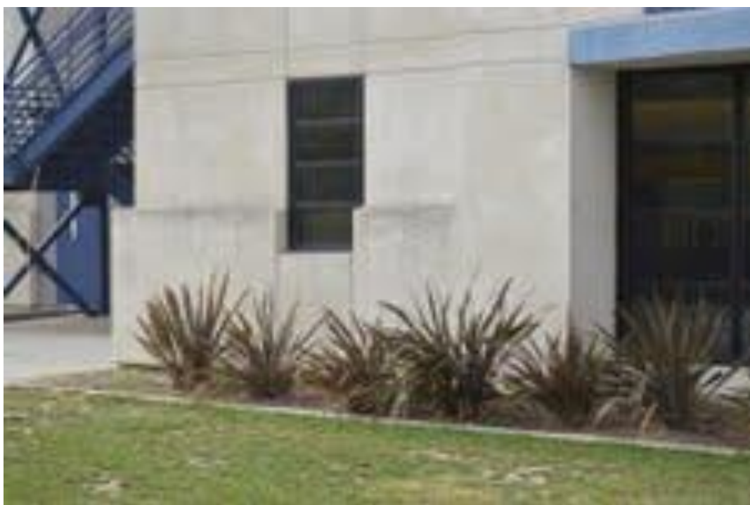
Control - Built in 2009. Not Treated. Not cleaned. Photo taken in 2013
