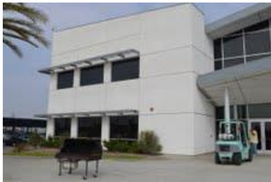
PURETi – Built in 2009. Treated. Never cleaned. Photo taken in 2013
