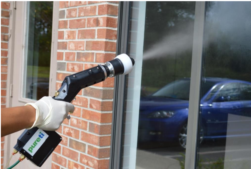
Applying on exterior glass
